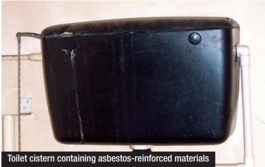
Toilet cistern containing asbestos-reinforced materials
